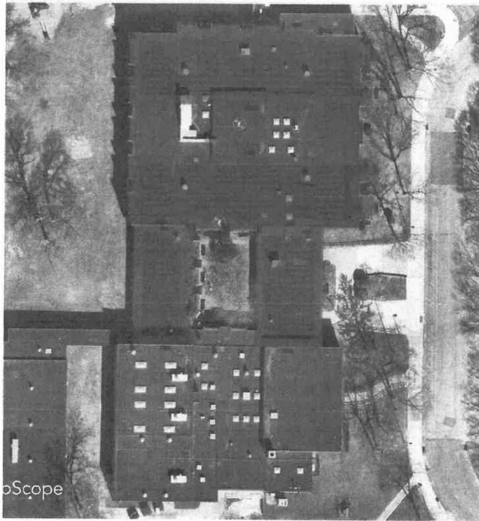
Cherokee Street Elementary School (155.2 kW)
